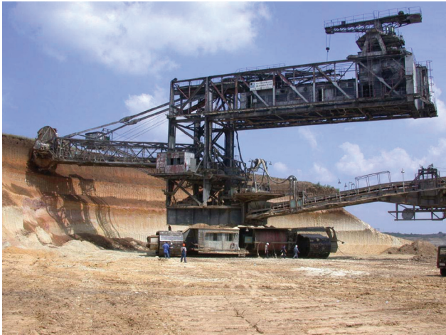
Figure 4 – Look of bucket-wheel excavator SRs 1200 24/4 (G2) before the accident appearance.
